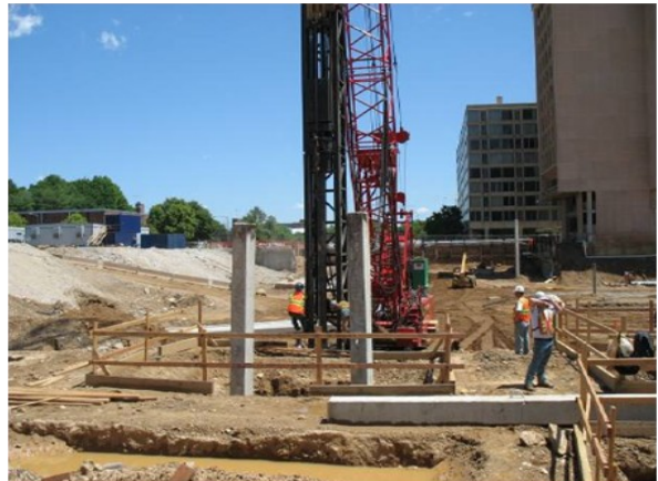
Driven Pile Inspection, Metro Water-front Station Development, DC
